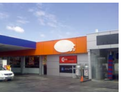
Mogas Heuley Petrol Station Adelaide, Australia tesa® ACX plus 70200
