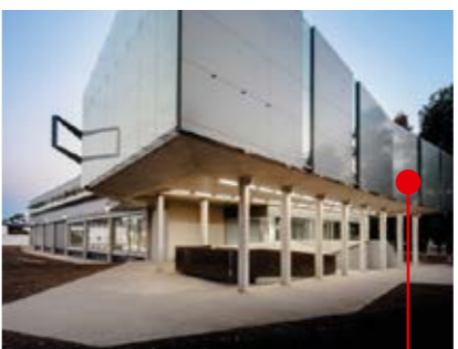
Federal Police Building Adelaide, Australia tesa® ACX plus 70200
