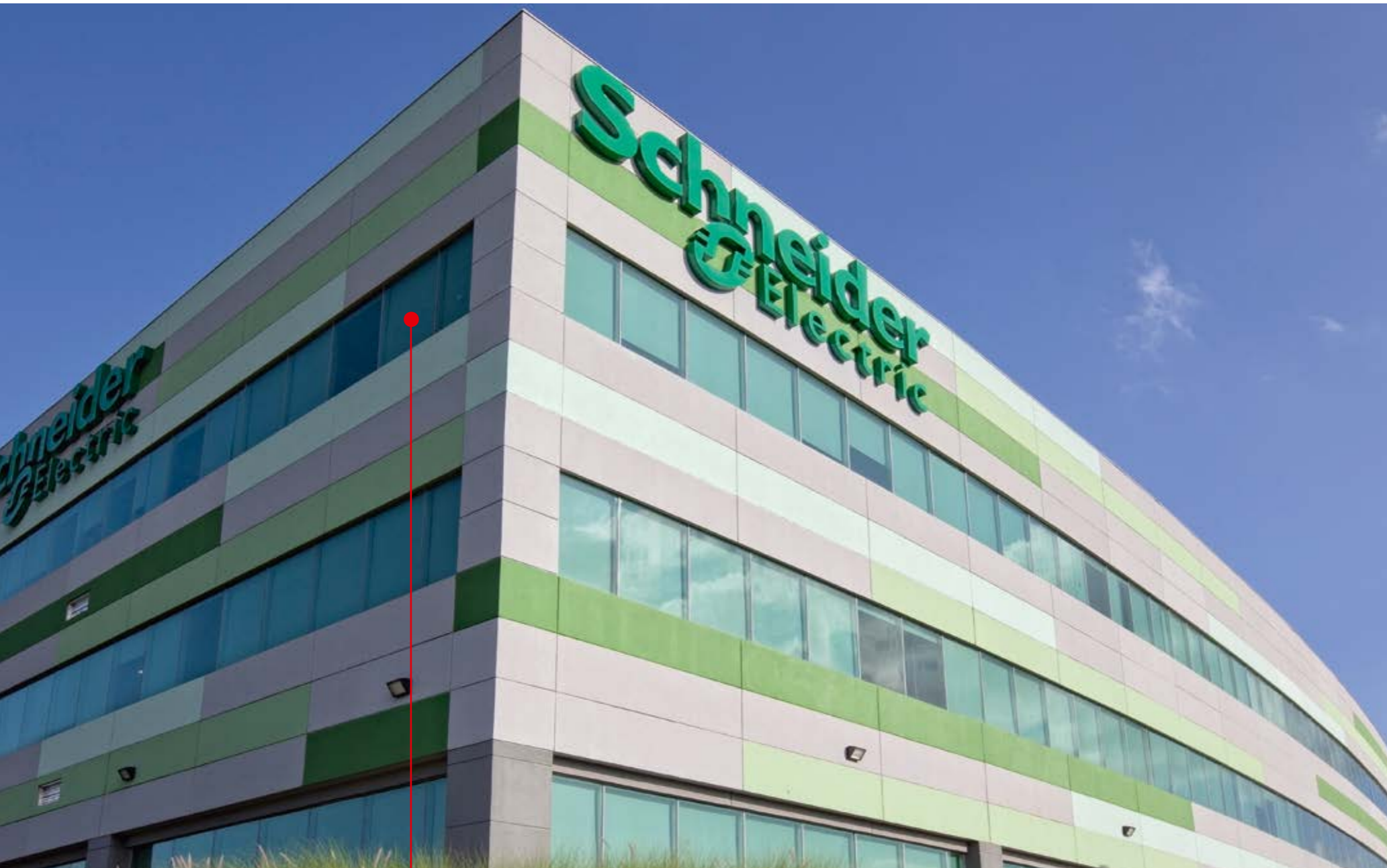
Schneider Building Montreal, Mexico tesa® ACX plus 70200
