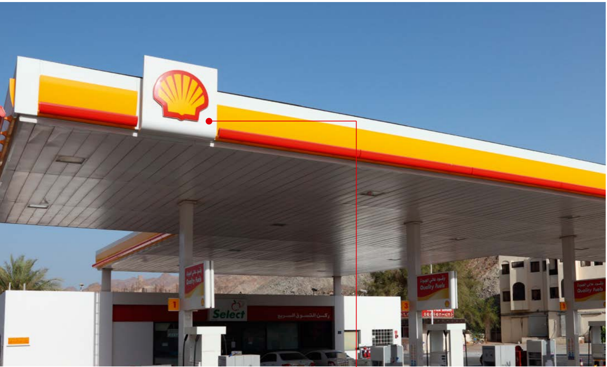
Shell Monolights Kuala Lumpur, Malaysia tesa® ACX plus 7074
