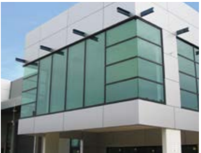
Industrial Complex Churolla, Australia tesa® ACX plus 70200
